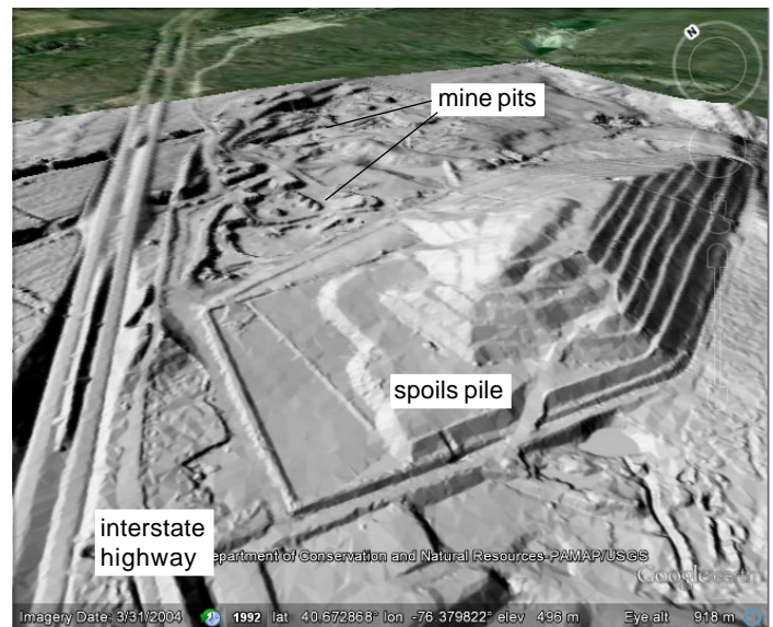
Shaded-relief Google Earth 3D tileset of a surface coal mine in eastern Pennsylvania. Terrain and shading created from Lidar DEM with 1-meter cell size. A large terraced spoils pile is in front of the shallow mine pits.
